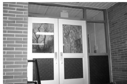
The District's door project has replaced aged, wooden doors at all schools with steel doors that meet fire code and are energy efficient.
