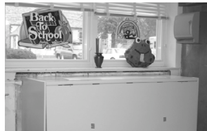
Aged, inefficient radiators and unit ventilators at VMS have been replaced with energy efficient heating system components.
