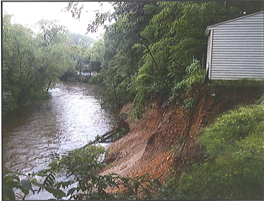
Figure 1. View of Existing Shed on Rear Lot of 15 Lakeshore Drive
