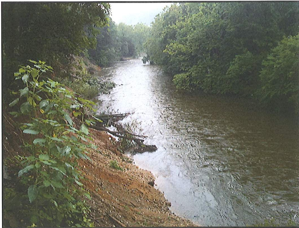
Figure 2. Downstream View of Ramapo River Stream Bank
