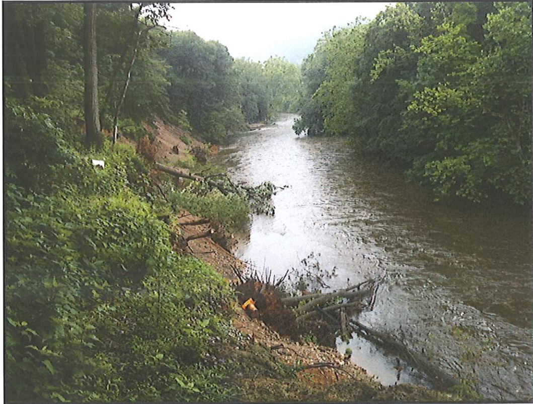
Figure 3. Additional Downstream View of Ramapo River Stream Bank
